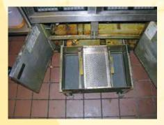
Insert the hold down ring and press it firmly into place. Finally, insert the crumb catcher.
